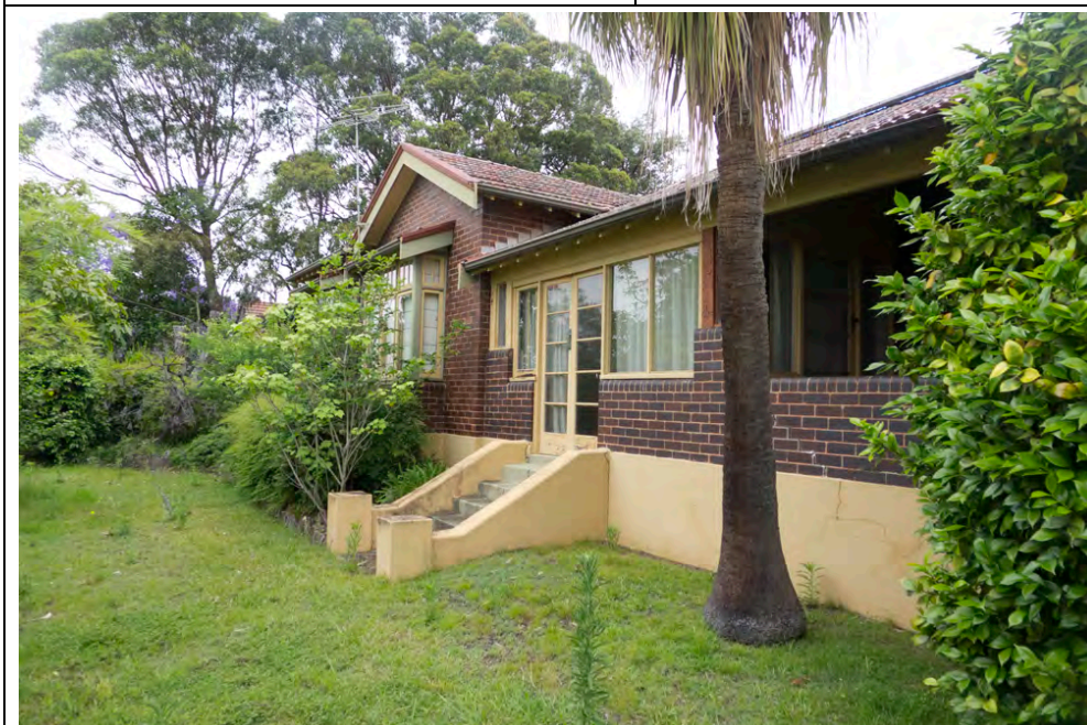
Figure 29: The western elevation of the house, showing the circa 1950s partial verandah enclosure to form a sunroom (centre) with the original western steps onto the verandah remaining.
