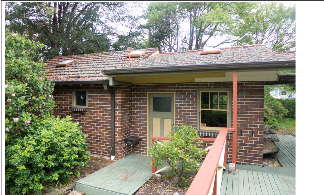
Figure 49: The western elevation of the modern garage (at left) and workshop (at right).
