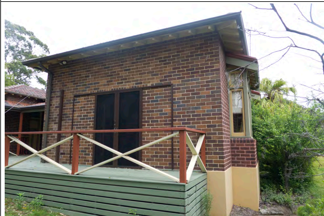
Figure 35: North-west corner of the house
