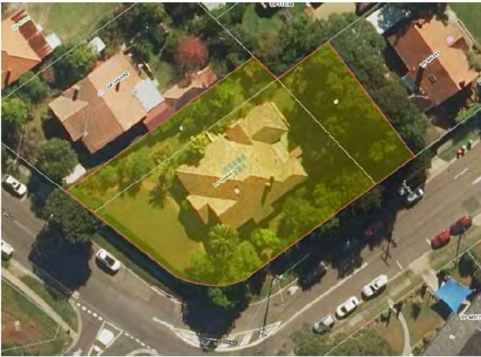
Figure 3: Aerial Photograph of the site (Source: Paul Davies Pty Ltd, Heritage Assessment Report p7)
