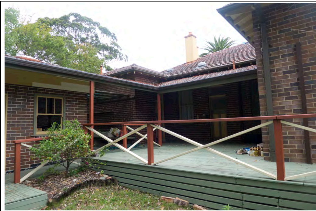
Figure 34: View of the rear (north elevation) of the house including a chimney, with the garage/workshop at left
