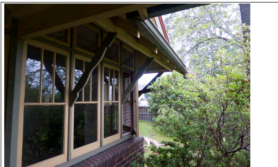
Figure 26: Detail of timber-framed casement bay windows with fanlights and window hood.
