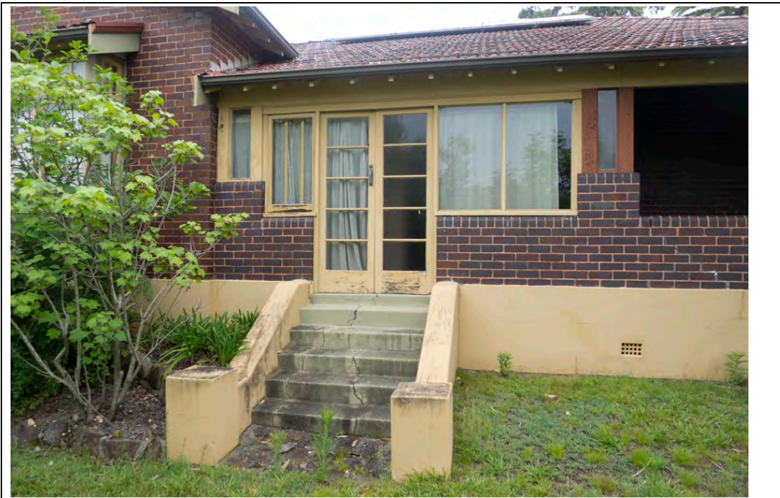
Figure 30: Detail of western verandah circa 1950s sunroom enclosure and original western steps onto verandah. Note cracking of stairs and brickwork in verandah wall to the right of photo.
