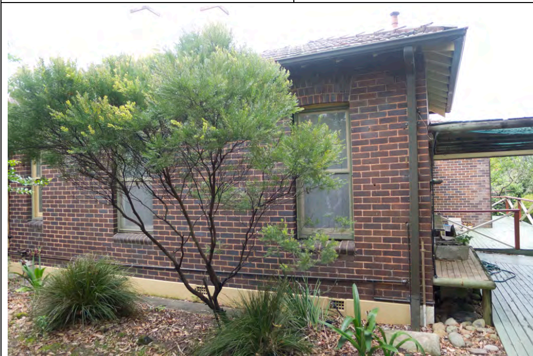
Figure 39: (Left) the north-eastern corner of the house. The two windows shown here are to the kitchen (left) and laundry (right)
