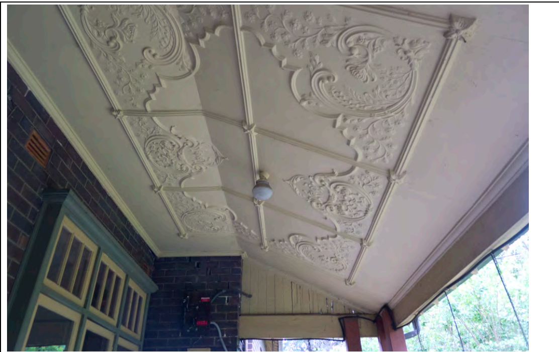
Figure 46: Decorative plaster ceiling to eastern verandah
