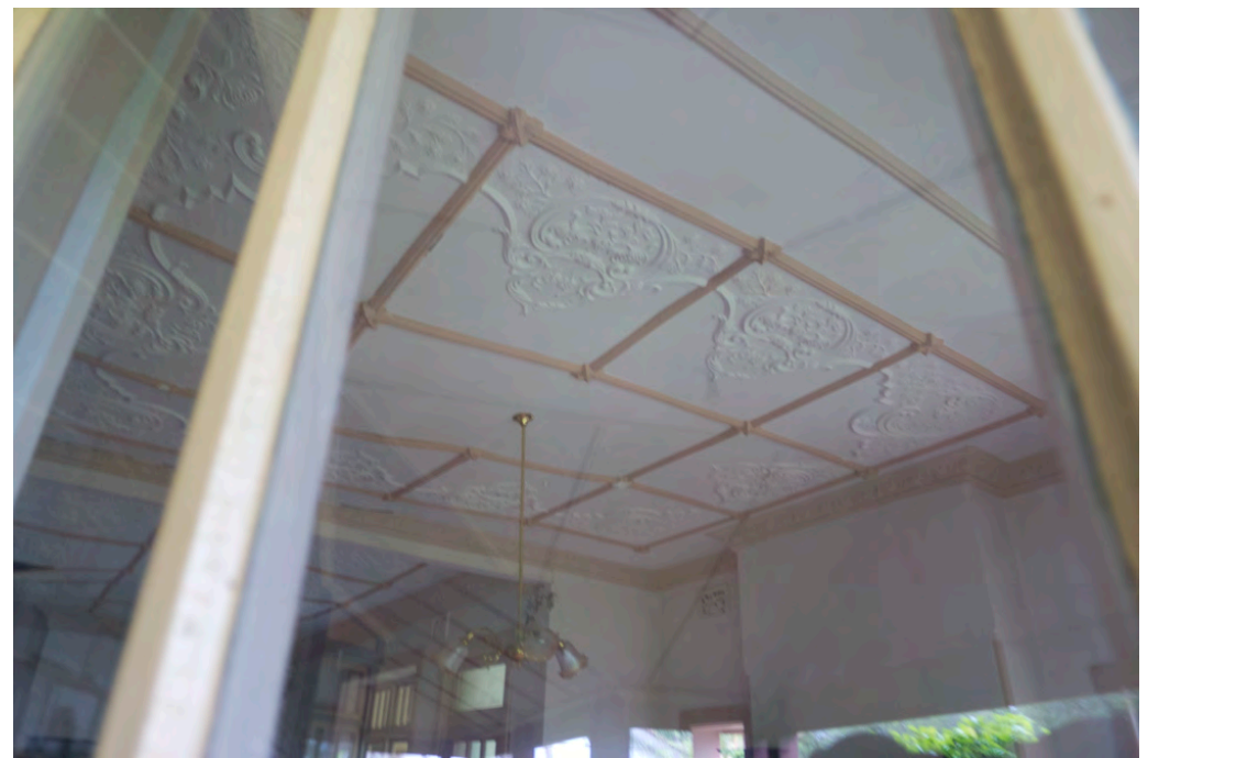
Figure 58: Loungeroom ceiling, taken through front bay window, November 2018
