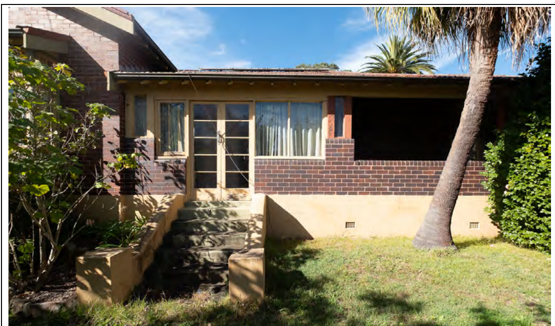
Figure 66: Sunroom to north-western elevation – enclosure of part of the side verandah. This alteration is easily reversible, with the original verandah steps in the foreground. May 2019.
