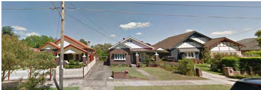
Figure 74: Houses at 17-21 Maxim Street, West Ryde Source: Image from Google Streetview
