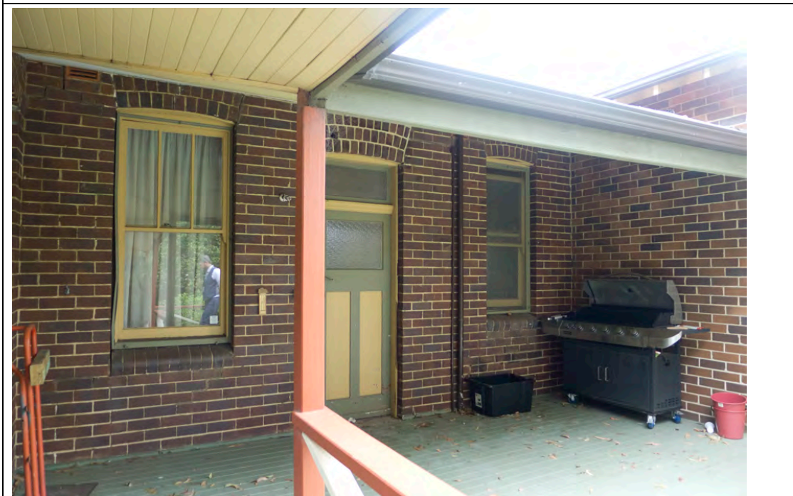
Figure 37: Central section of the rear (north) elevation
