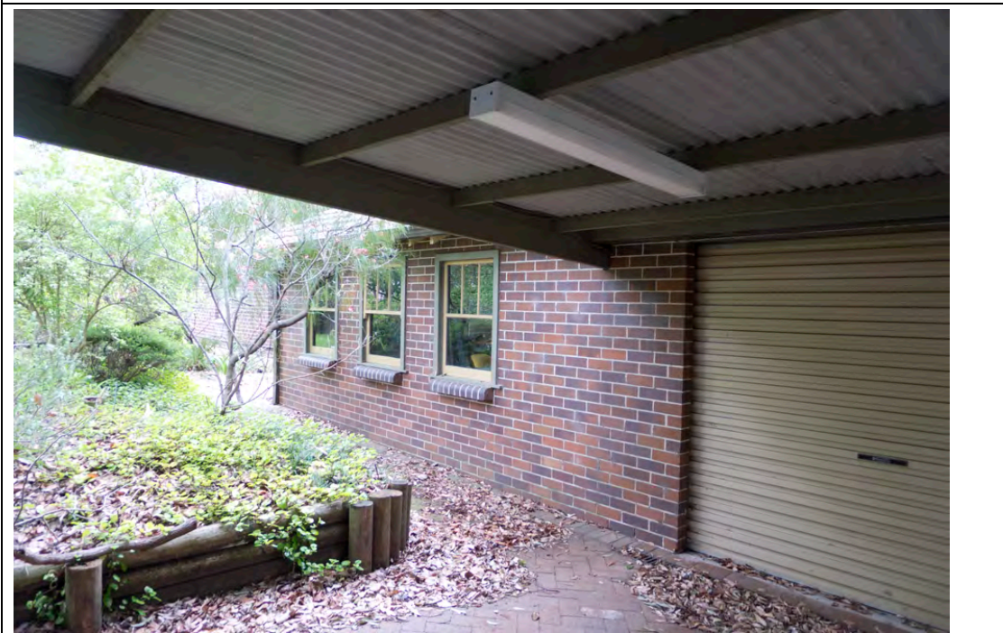
Figure 47: The eastern elevation of the carport and garage/workshop off Florence Avenue
