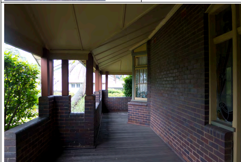
Figure 25: View along front verandah to the west, showing complex ceiling form and bay window.
