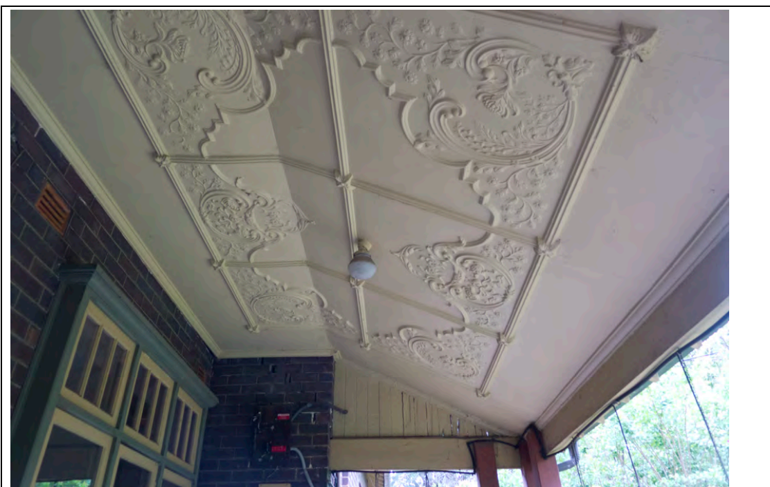
Figure 46: Decorative plaster ceiling to eastern verandah
