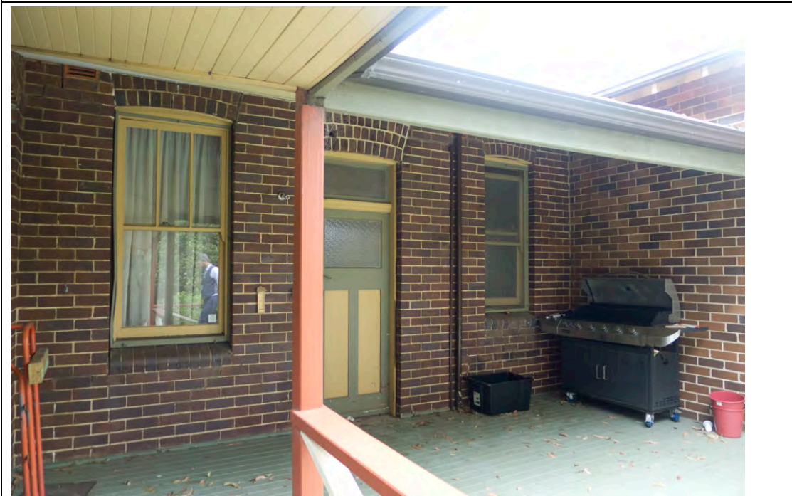
Figure 37: Central section of the rear (north) elevation
