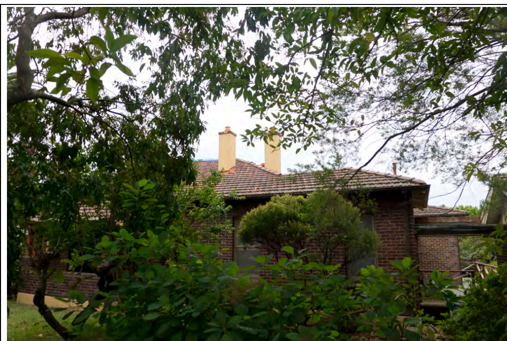
Figure 40: View of the rear of the house from the east, showing the chimneys to the rear of the dining room and to bedroom 3
