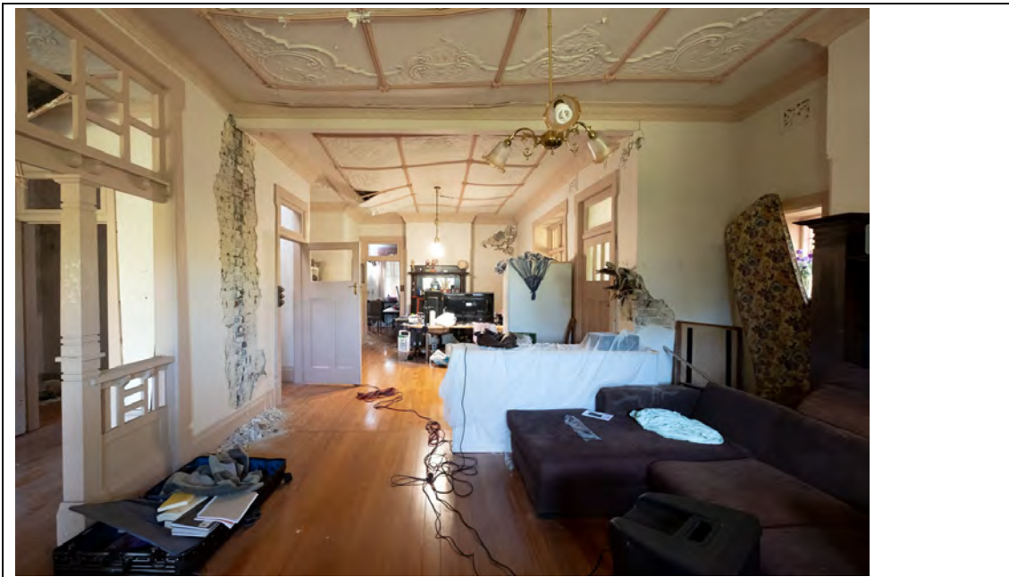
Figure 56: View of lounge room and dining room looking north, May 2019. Note damage to walls and collapsing ceilings
