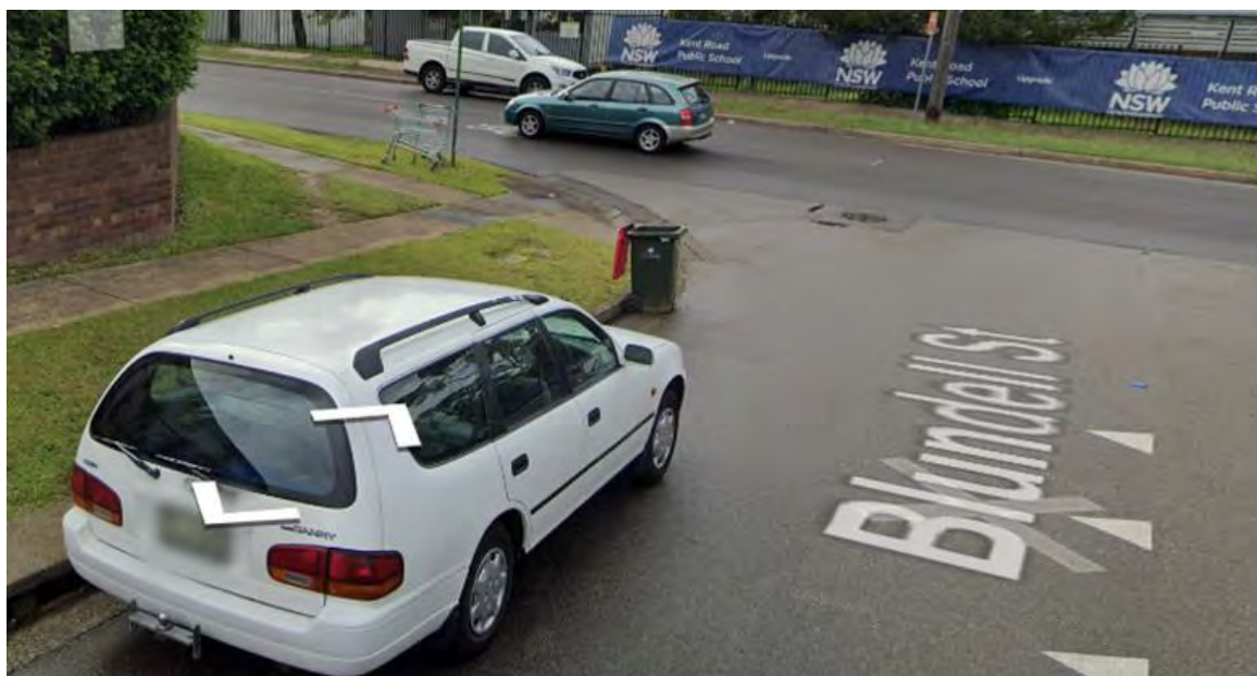
Figure 4: Missing No Stopping Restrictions
