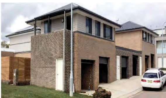
Example of an affordable 'fonzie flat' in the Potts Hill Community Housing precinct in Bankstown
