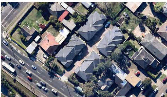
A key issue for villa developments is the extent of site coverage and lack of vegetation (Victoria Road, Ryde)
