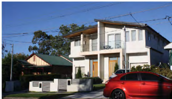
The varied front setback on this dual occupancy helps to create interest and break the bulk of the built form
