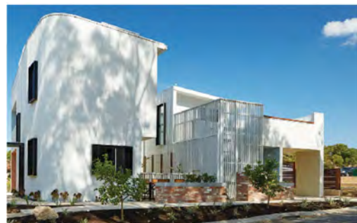
Example of a manor house on a corner lot (Source: Medium Density Housing Code)
