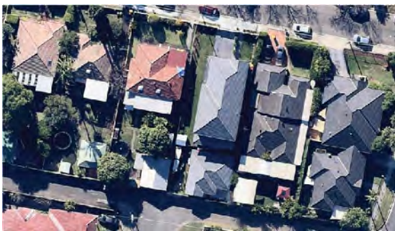
Aerial view of a recent secondary dwelling accessed off Annie Lane, West Ryde
