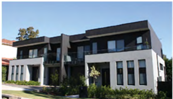
Instead of stepping, maintaining the same floor level for both dwellings increase the development's bulk
