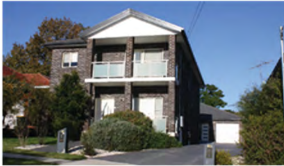
Example of a dual occupancy in the Ryde LGA with one building behind the other
