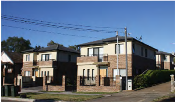
Townhouse development located in Denistone with on grade shared access to car parking
