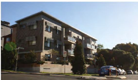
A more traditional (older) 3 storey low rise apartment building in Top Ryde is a frequent typology across Sydney
