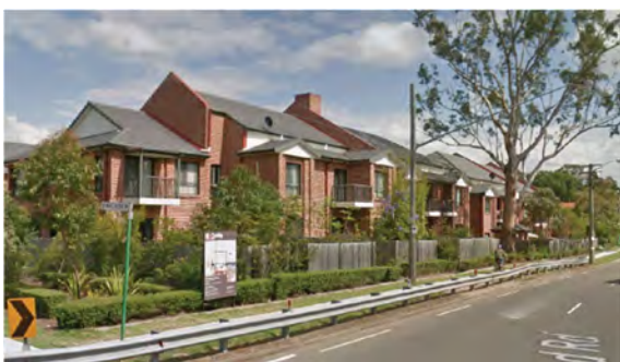
The use of pitched roofs and articulation of the facade along the street helps to break the bulk of the built form
