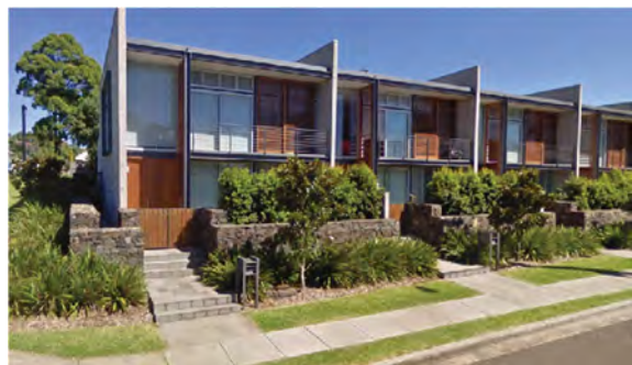
These strata titled terraces in Kiama successfully address the street with parking to the rear
