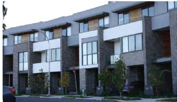
Front loaded terrace houses in Putney Hill with a variety of materials, windows and balconies
