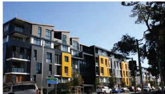
This development in Meadowbank applies a 4+2 and 4+1 built form (4 storeys plus 1-2 upper storeys))
