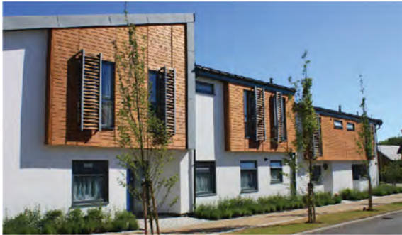
An example of a low-rise apartment development in Newhall UK
