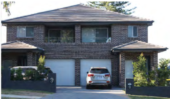
Mirrored dual occupancies often increase the visual bulk of the built form when viewed from the street
