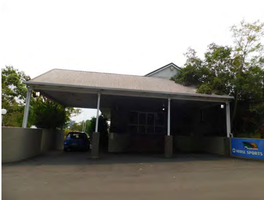
Figure 25: Part of south-eastern elevation of the altered 1960s club building
