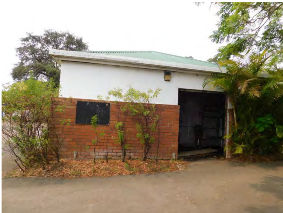
Figure 29: RUFC building to the south of the club building
