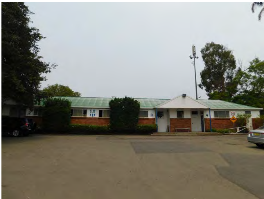
Figure 32: RUFC Building to the north-east of the club building
