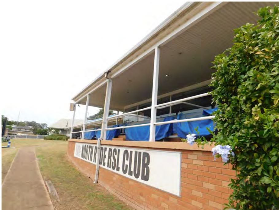
Figure 24: North-western elevation of the altered 1960s club building
