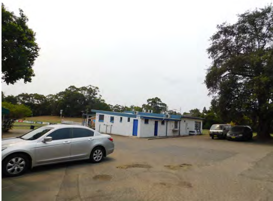
Figure 31: Eastern Rugby Amenities block to the north-east of the club building
