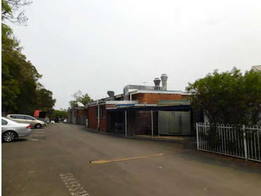
Figure 27: View along the south-eastern elevation of the club building looking towards the carparking area
