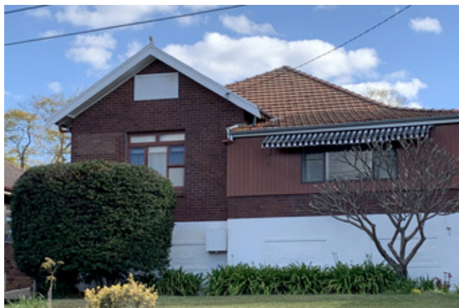
Reconstruction of window hood, reinstatement of casement window and leadlight glass in traditional pattern.
