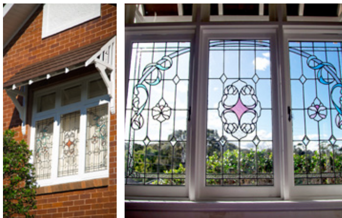
Reconstruction of window hood, reinstatement of casement window and leadlight glass in traditional pattern.
