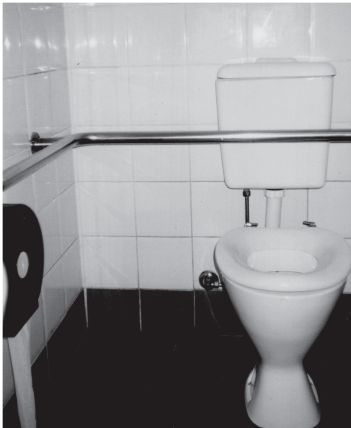
Figure 9.2.04 Toilet centreline is more than 460 mm from wall, putting paper and the handrail out of easy reach
