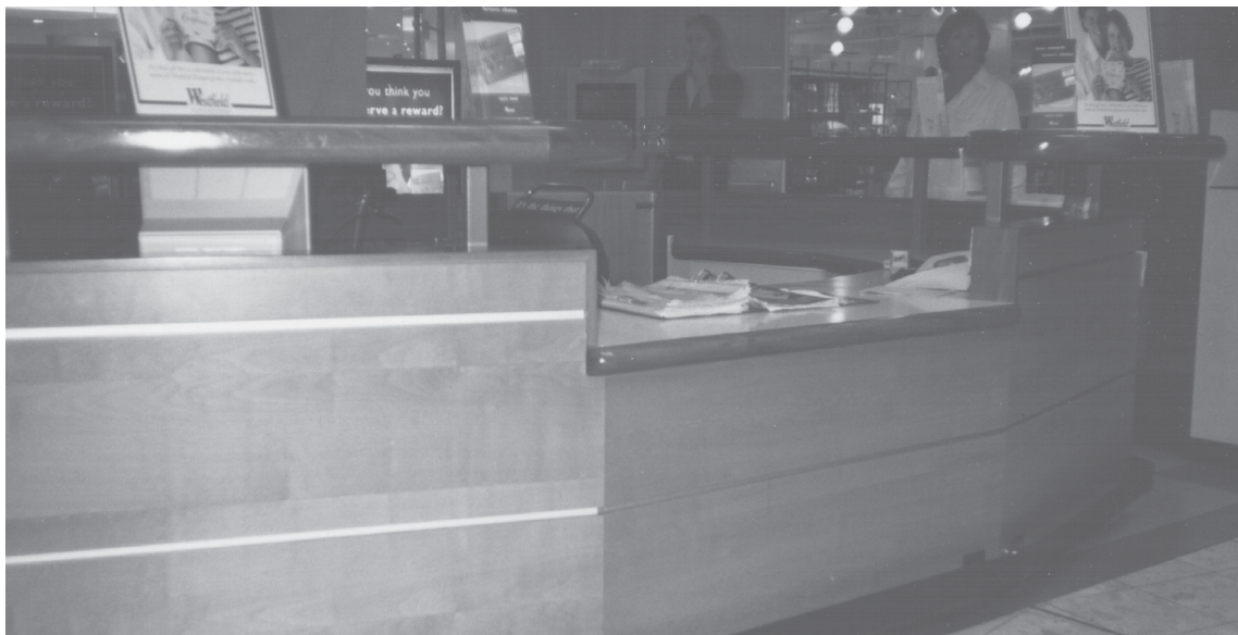
Figure 9.2.06 Lower counter area is good for wheelchair users but lack of space under counter means it cannot be used to write on
