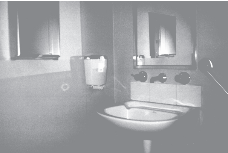
Figure 9.2.05 Towel dispenser is too high above floor and soap dispenser is too close to corner. Mirror is too high for wheelchair users.
