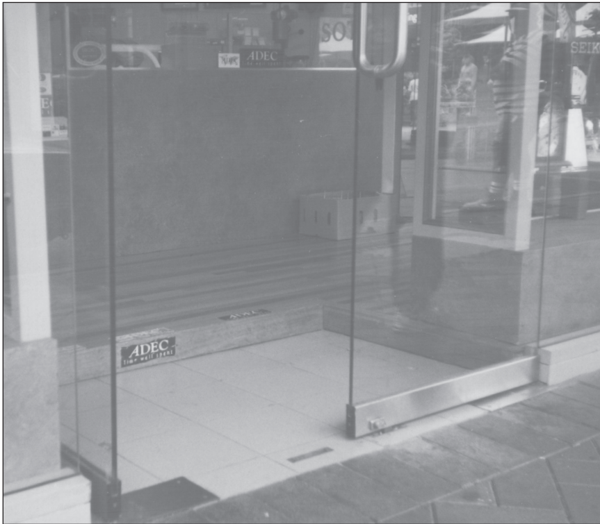
Figure 9.2.02 The false floor prevents access and the doors are less than 960mm in width
