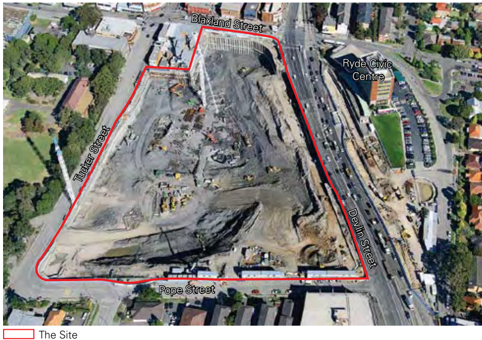
Figure 4 – Aerial photograph of the current construction works on the site (May 2008)
