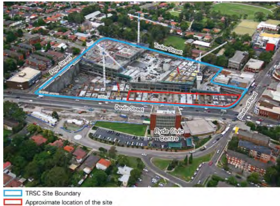
Figure 3 – Aerial photograph of the construction works on the TRSC site (November 2008)
