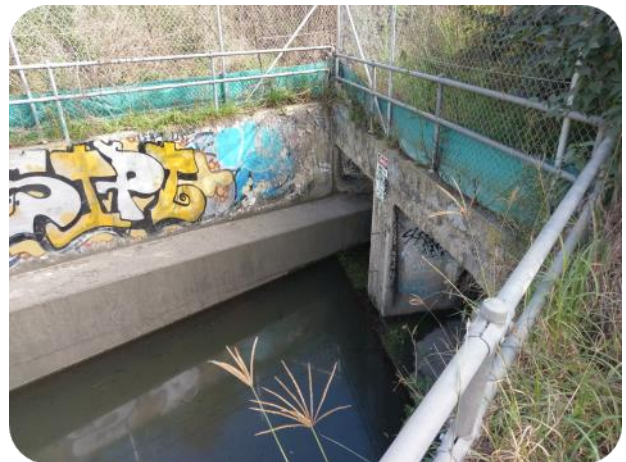
Figure 31 Porters Creek @ Main Branch facing downstream
