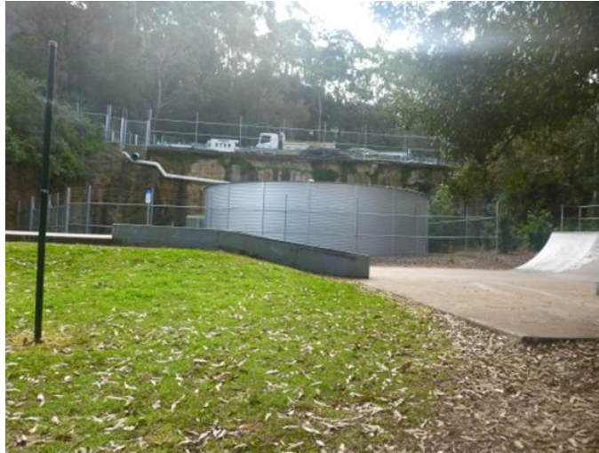
Figure 12-6: Existing Stormwater Tank at Blackman Park
