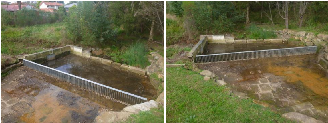
Figure 12-7: Existing Bio-Retention System at Santa Rosa Park (Shrimptons Creek)
