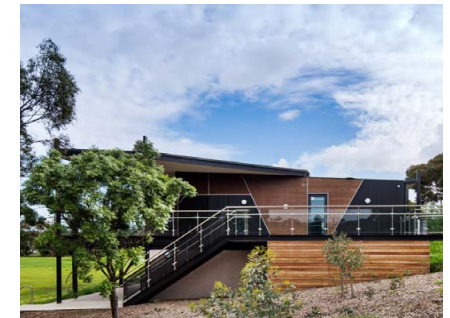
Aberfeldie Park Pavilion by JM Architects - two-storey building constructed into slope and providing access from both sides
