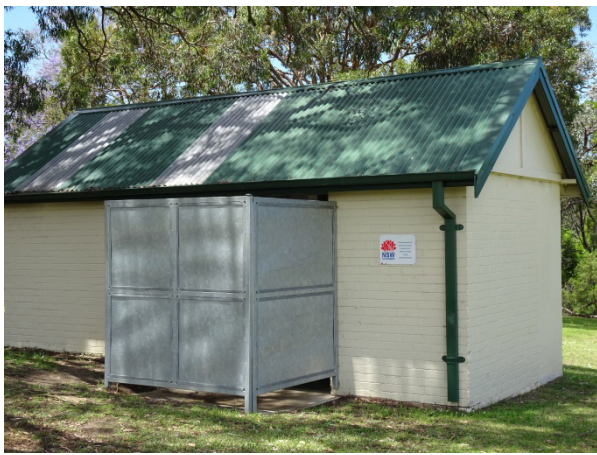
Toilets at Tyagarah Park
