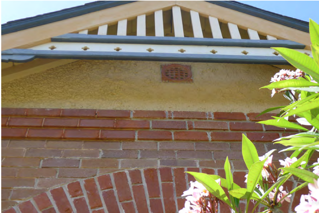
Figure 28: Detail of north gable end, showing decorative timber flying gable end, roughcast stucco, polychrome brickwork and terracotta vent
