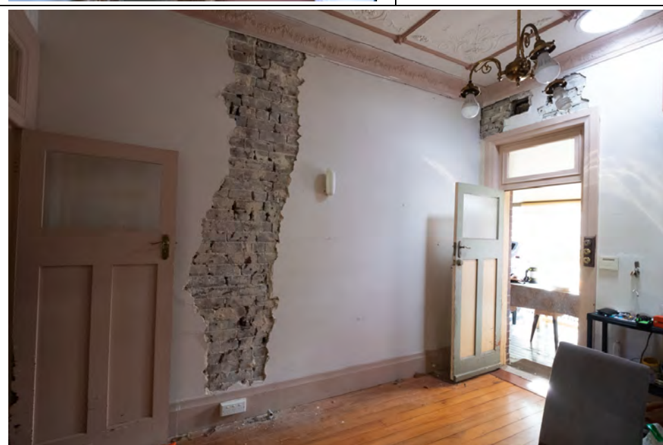
Figure 61: Breakfast room wall damage. May 2019.
