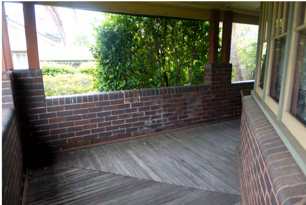
Figure 27: Detail of south-western corner of the return verandah showing brick balustrade, timber posts and timber verandah floor
