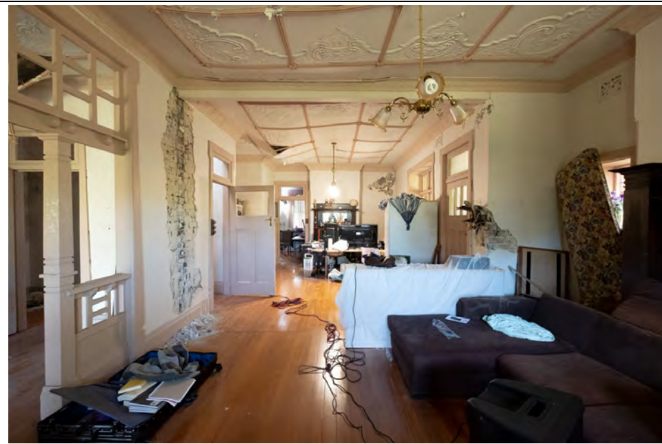
Figure 56: View of lounge room and dining room looking north, May 2019. Note damage to walls and collapsing ceilings
