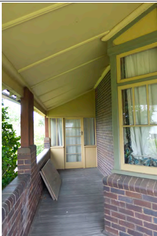
Figure 28: (Left) View along the western side of the return verandah showing circa 1950s infill at the northern end of the verandah. According to the real estate floor plan, this partial verandah enclosure is a sunroom, however the original steps onto the verandah on the western side of the house remain (see below).
