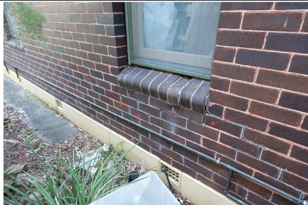
Figure 64: Minor cracking evident on north-western wall (arrowed). May 2019
