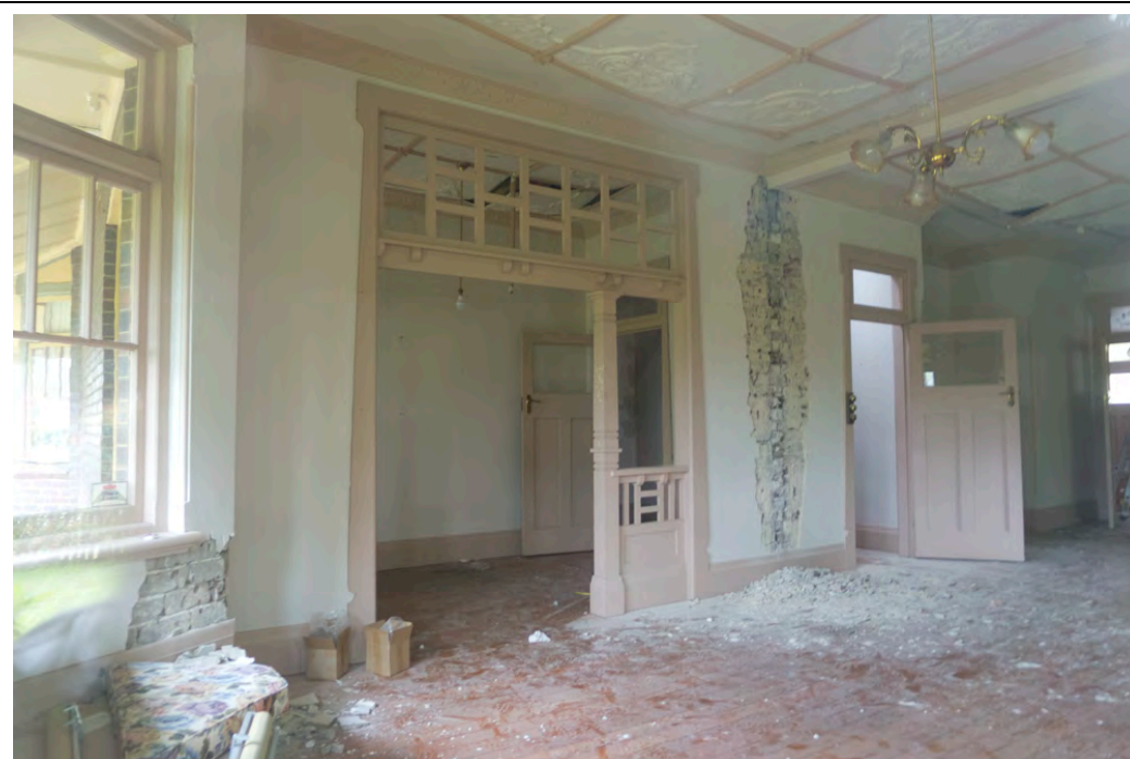
Figure 59: View of wall between loungeroom and hallway (foyer). Note the damage to the wall plaster is a result of illegal building works which occurred prior to the IHO on the site. Taken November 2018
