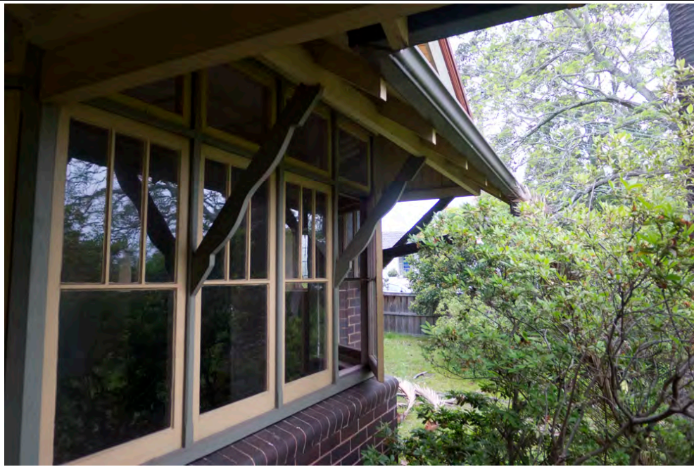
Figure 26: Detail of timber-framed casement bay windows with fanlights and window hood.
