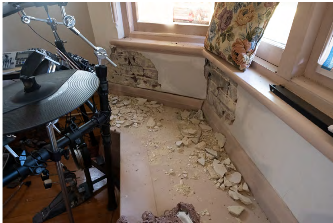
Figure 63: Damage to plasterwork near front bay window of the lounge room. May 2019
