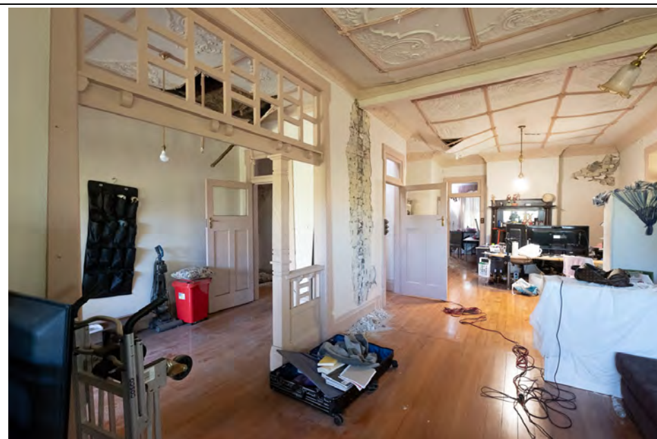
Figure 53: View of lounge room to hall, note wall damage and collapsing ceilings.
