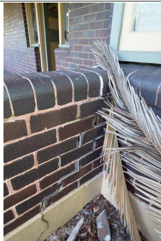
Figure 64: Minor cracking evident on north-western wall (arrowed). May 2019
