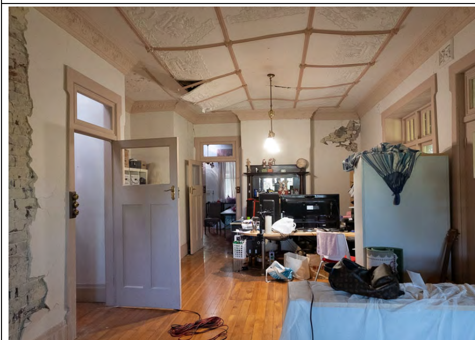
Figure 55: Same view of the dining room looking north towards the rear of the house, May 2019, noting ceiling and plasterwork damage.
