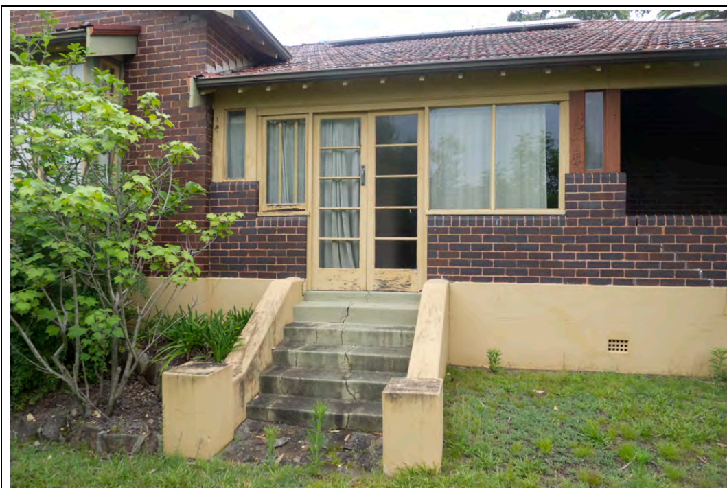
Figure 30: Detail of western verandah circa 1950s sunroom enclosure and original western steps onto verandah. Note cracking of stairs and brickwork in verandah wall to the right of photo.
