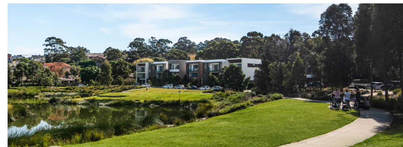
Example of low-rise medium-density housing (Terraces), Putney Hill
