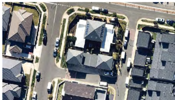
Aerial view of two of the 'fonzie flats' (see adjacent photo 05) addressing Rowe Lane, Potts Hill
