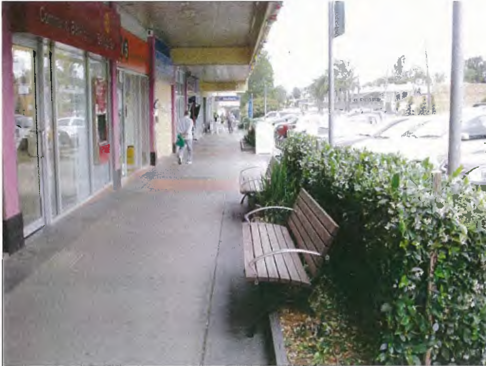
North side of Coxs Rd showing coloured concrete and both granite and clay pavers.
