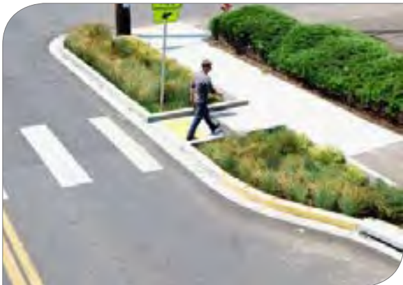
Using bulb-outs or curb extensions for traffic calming and provide ease for pedestrian crossing (source: U.S. Environmental Protection Agency)
