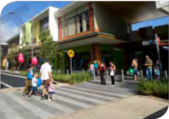
Using raised crossing with surface treatment for traffic calming (source: Bylett and Associates)
