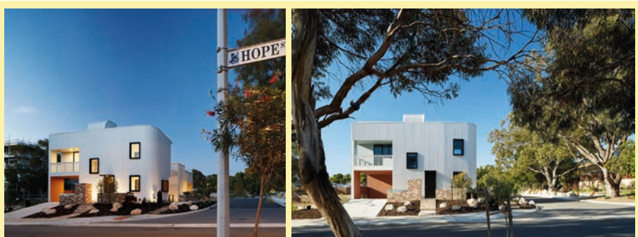
White Gum Valley, David Barr Architects
