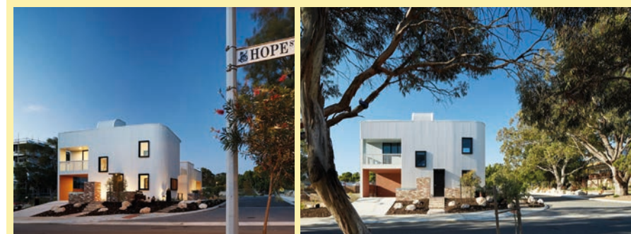
White Gum Valley, David Barr Architects
