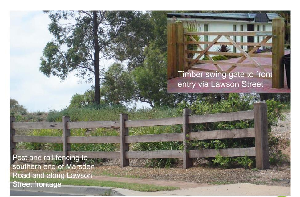
Fencing: Post and Rail timber fencing
