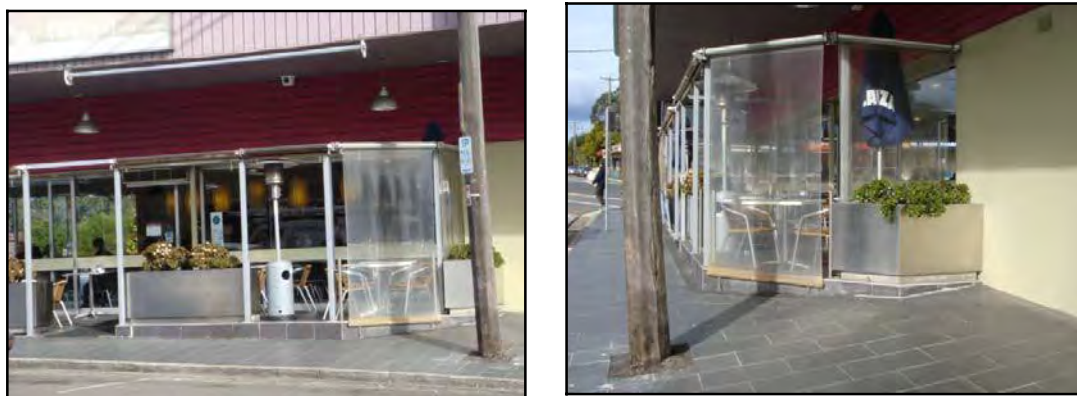
Figure 2 Example of minor works to the footpath area ensuring a level platform for the outdoor dining area. Diners are protected from the change in level by trellis balustrading and planter boxes.
