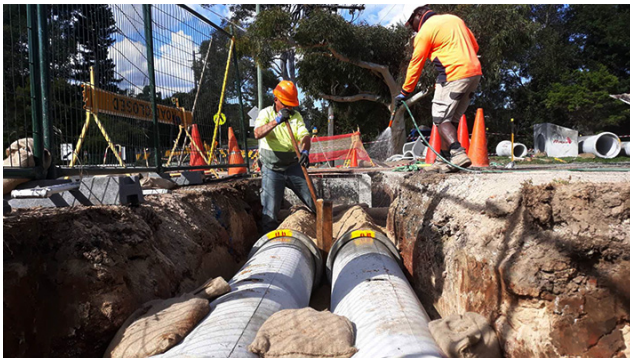
Example stormwater drainage works in progress
