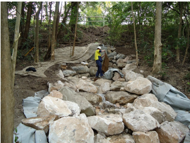
Example rock lined channel works in progress (Source: Soil Conservation Services)
