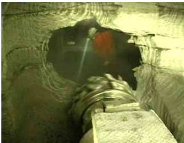
* The West Ryde Stormwater Tunnel was completed during the year.
