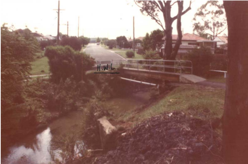
Photo A1.9 Photo taken of footbridge with Lucinda Road in background (Ryde City Council photo 'S26')
