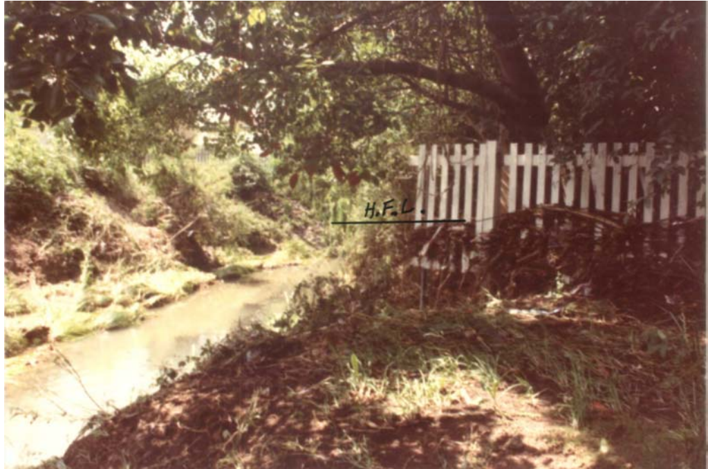
Photo A1.11: Debris deposited against Bridge Road property fence, on south bank of Shrimptons Creek. (Property has since been purchased and house, etc demolished).
