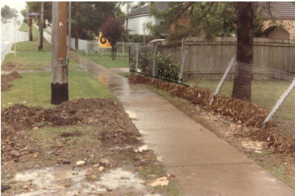
Photo A1.10: Debris deposited at property on corner of Herring Road and Lucinda Road, looking east along Herring Road. (Ryde City Council photo 'S29')
