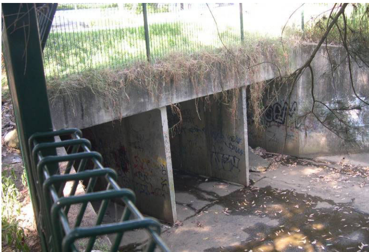
g. Entrance to three cell box culvert conduit upstream of Waterloo Road
