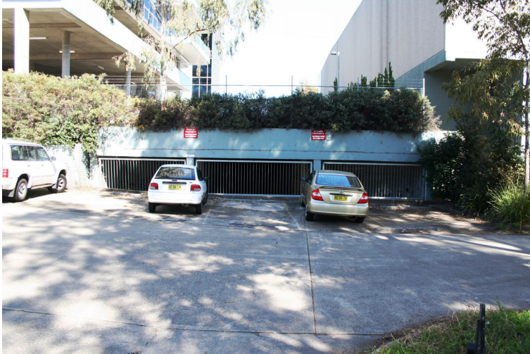
d. Culvert surcharge outlet at downstream end of Officeworks
