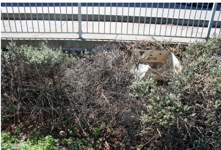
c. Blocked culvert inlet at Officeworks
