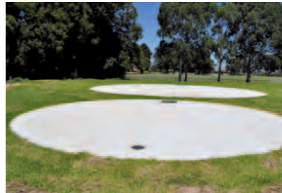
Epping Oval Stormwater Harvesting Project – Storage Tanks – Photo: Neil Keraunos.
