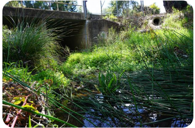
Figure 11 Shrimptons Creek at Kent Rd facing downstream
