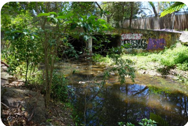
Figure 31 Buffalo Creek Upstream of Burrows Park
