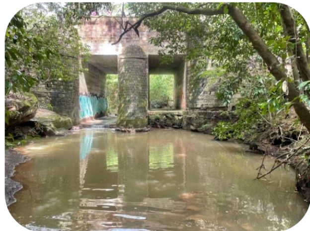
Figure 36 Porters Creek Core Site looking upstream
