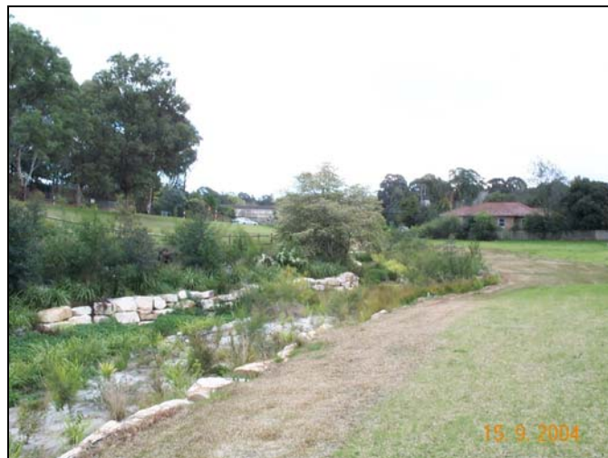
Figure 13: Archer Ck facing upstream to restoration works.
