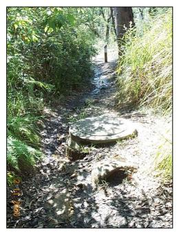
Figure 10:Leaking pipe along walking track to Terrys Ck site.
