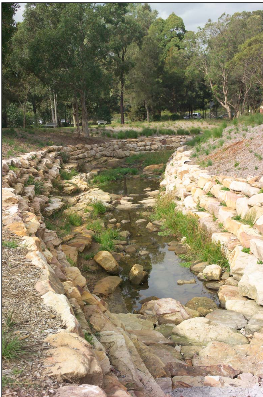
Figure 2 Archers Creek in Autumn 2008 showing completed rehabilitation work
