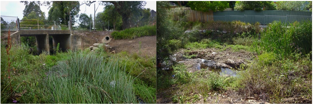
Figure 7 Shrimptons Creek, spring 2013, Bridge St (L) and Quarry Rd (R)
