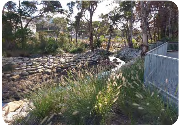
Figure 34 Porters Creek at Wicks Road
