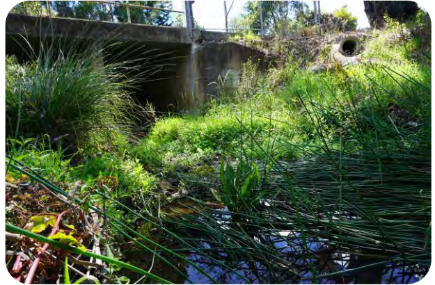
Figure 12 Shrimptons Creek at Bridge Road facing downstream
