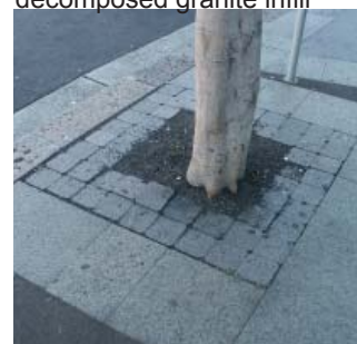
Granite setts terrabond infill
