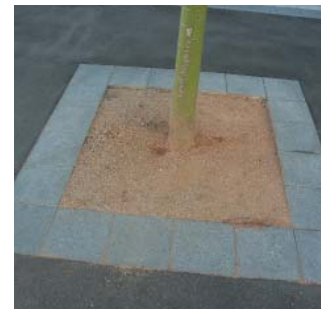
Paving surrounds with decomposed granite infill
