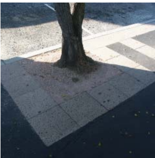
Paving surrounds with decomposed granite infill
