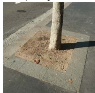
Paving surrounds with decomposed granite infill
