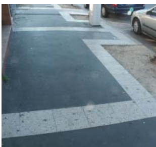
Pebblecrete paving trim + banding with bitumen infill
