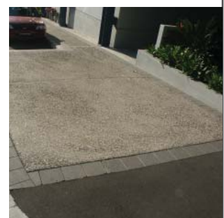
Granite paving with exposed aggregate concrete infill
