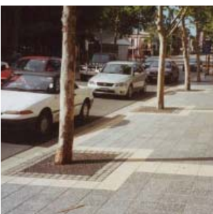
Granite setts terrabond infill
