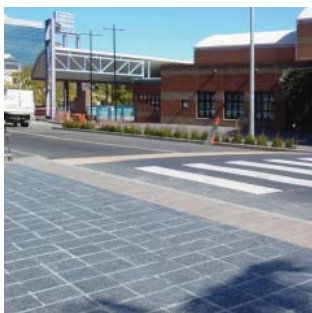
Coloured bitumen threshold
