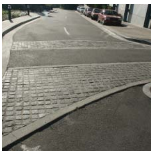
Granite setts as threshold
