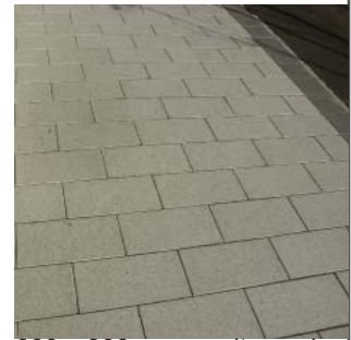
600 x 300mm granite paving
