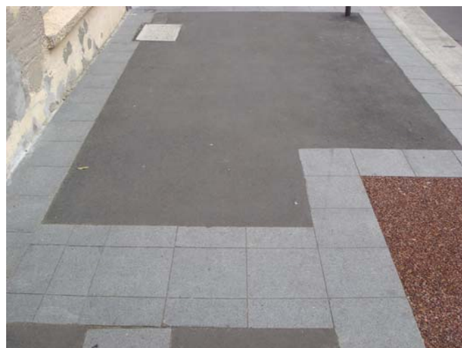
Asphalt with granite banding
