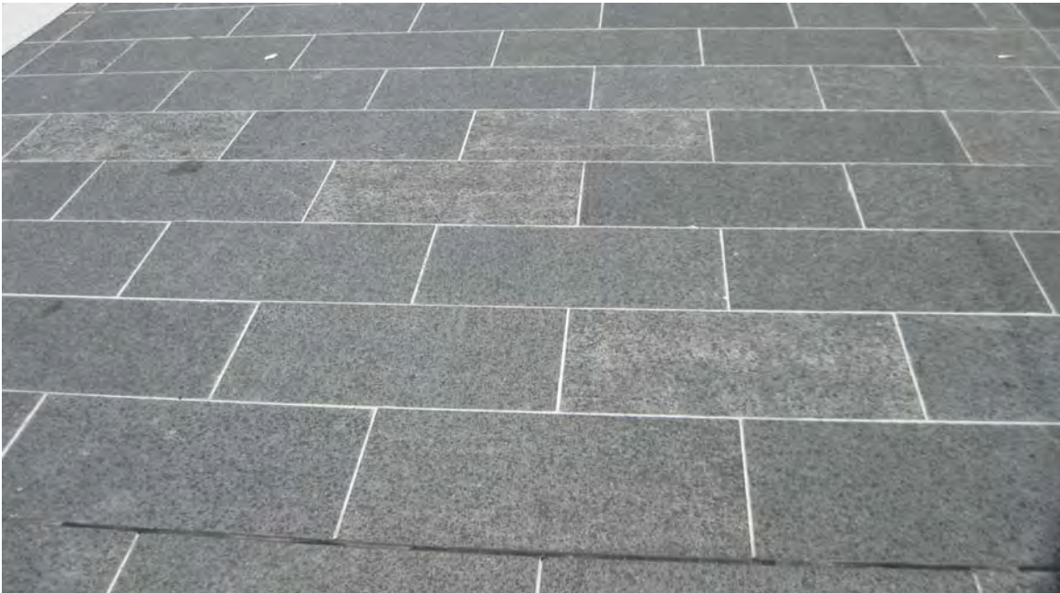
Granite Paving (Paving Type 2) - Meadowbank
