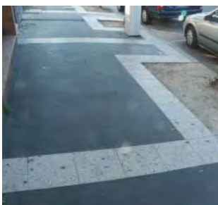
Pebblecrete paving trim + banding with bitumen infill
