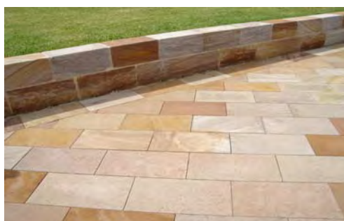
Sandstone paving 600 x 300 x 100mm (Ryde Wharf Park).
