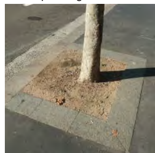
Paving surrounds with decomposed granite infill
