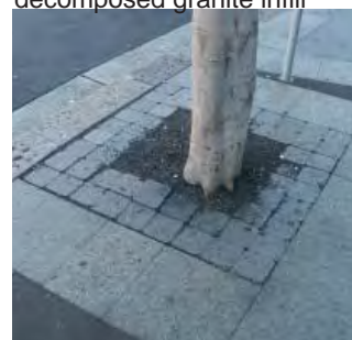
Granite setts terrabond infill
