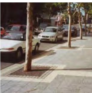
Granite setts terrabond infill
