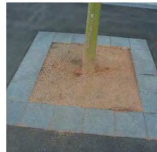
Paving surrounds with decomposed granite infill
