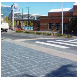
Coloured bitumen threshold
