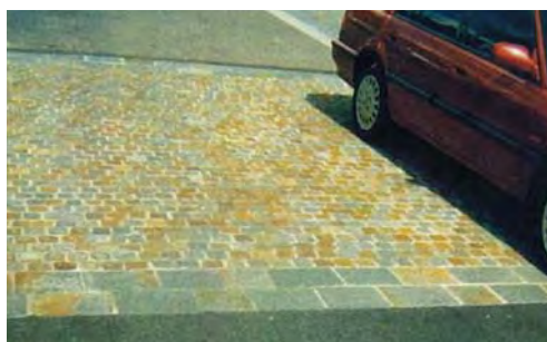
Australian porphyry stone for thresholds.
