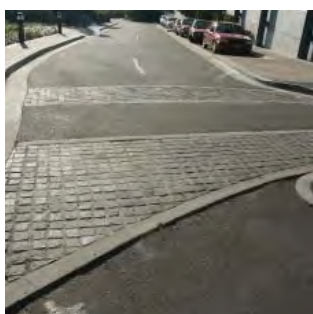
Granite setts as threshold
