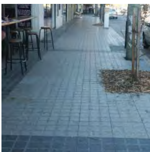
Granite paving with textured finish
