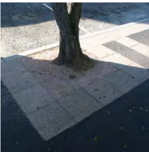
Paving surrounds with decomposed granite infill
