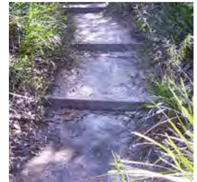
Track features - sleeper step and runs with sand or compacted fill treads.
