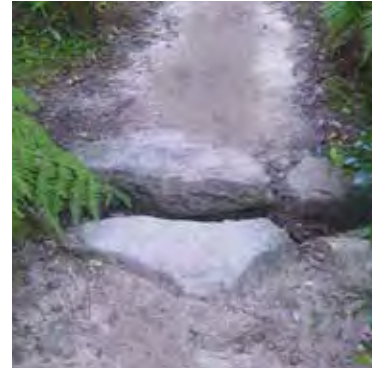
Track features - rock lined box drain / gutter.
