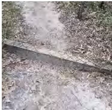
Track features - stormwater management using a sleeper water bar.
