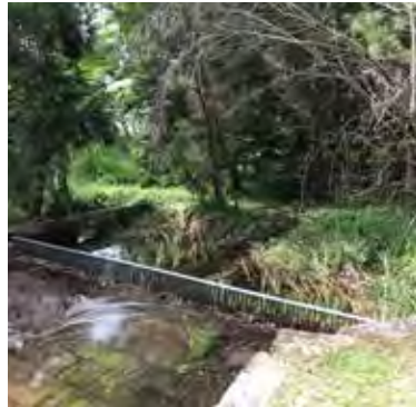
Existing trash rack and bio retention basin at the head of Strangers Creek.
