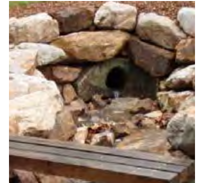
Rock lined headwalls and drainage lines to stormwater water outlets to manage erosion, before flowing to planted bio swales.
