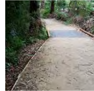
Accessible park path of crushed sandstone or compacted gravel with timber edge boards.
