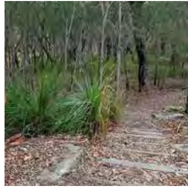
Track features - stepped path at an angle to the slope to manage drainage flows.
