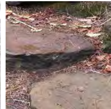
Track features - landing tread stone to armour track and prevent wearing from use.
