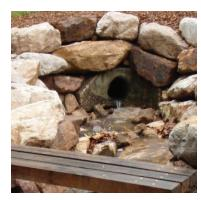
Rock lined headwalls and drainage lines to stormwater water outlets to mange erosion, before flowing to planted bio
