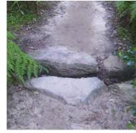
Track features - rock lined box drain / gutter.
