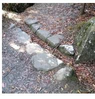
Track features - stormwater management using a stone gutter / box drain.
