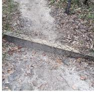
Track features - stormwater management using a sleeper water bar.
