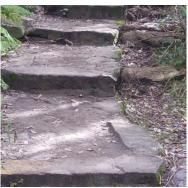
Track features - stone step and Track features - steps cut into runs with compacted fill treads. insitu rock.
