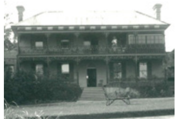
Brush Farm House 1910 Source: City of Ryde
