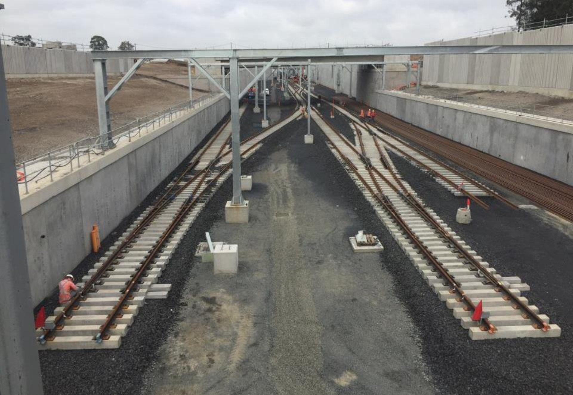
Approach to Cudgegong Road Station
