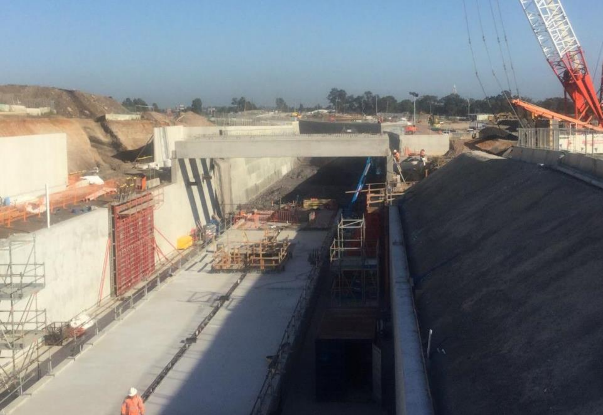
Bella Vista Station
