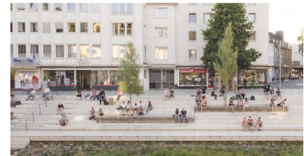
Precast concrete and planting areas to form Amphitheatre Seating Steps
