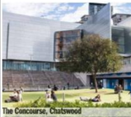
The Concourse, Chatswood
