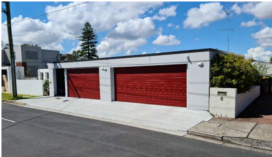
Figure 5: Adjoining dwelling situated at 4 Shackel Avenue, as viewed from Shackel Avenue
