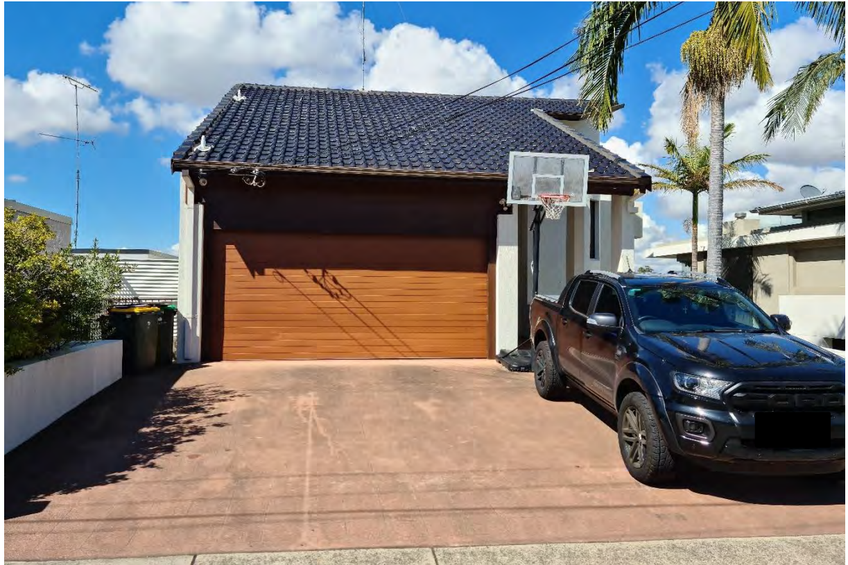
Figure 3: Existing dwelling on site subject to the proposed alterations and additions
