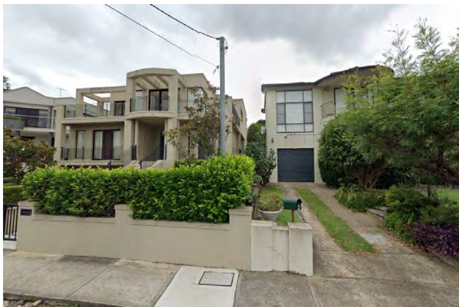
Figure 6: Dwellings situated at 3 Shackel Av (right) & 5 Shackel Av (left), as viewed from Shackel Avenue
