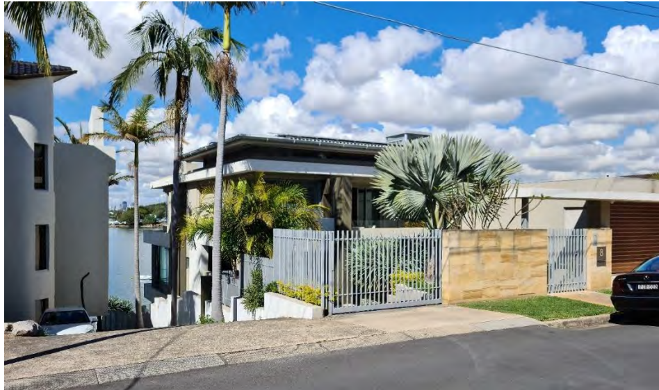
Figure 4: Adjoining dwelling situated at 8 Shackel Avenue, as viewed from Shackel Avenue
