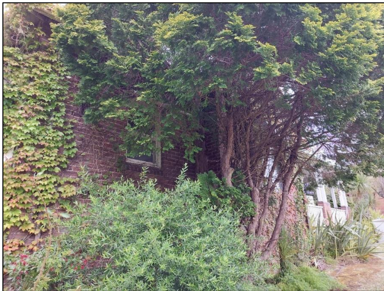
Figure 6 – Photograph of the Wentworth Road front elevation
