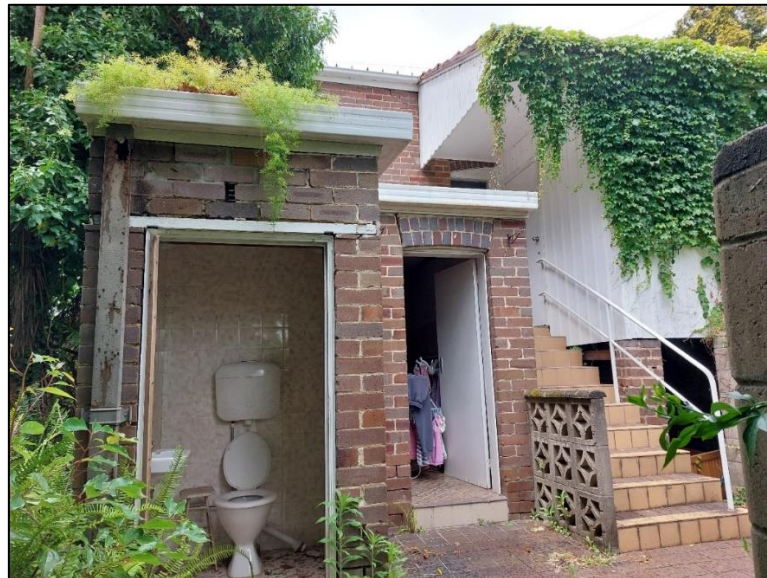
Figure 9 – Rear elevation of the existing dwelling
