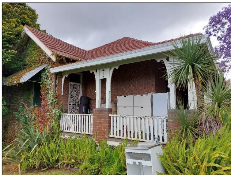
Figure 4 – Photograph of the Wentworth Road front elevation
