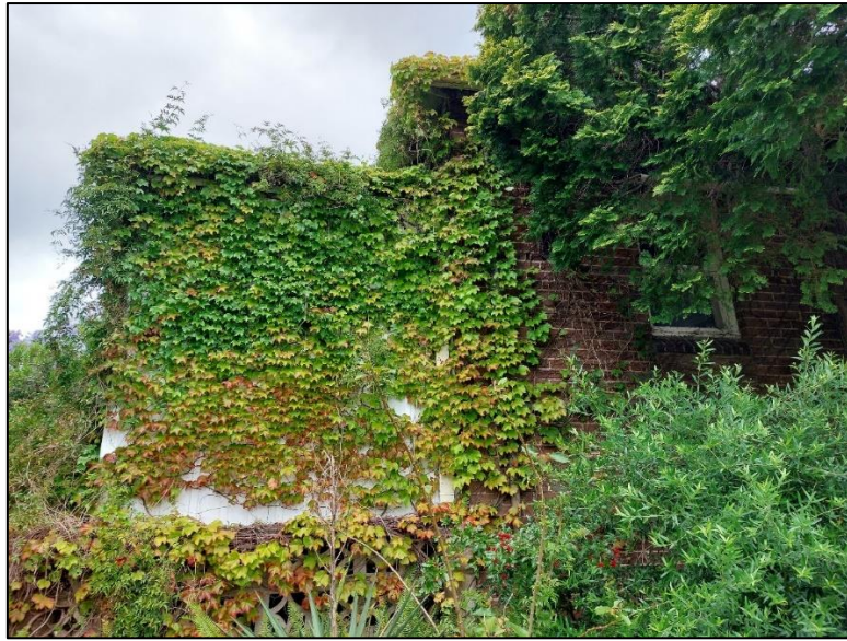
Figure 5 – Photograph of the Wentworth Road front elevation
