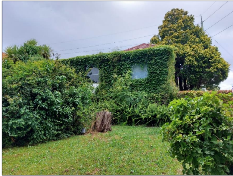
Figure 8 – Rear elevation of the existing dwelling
