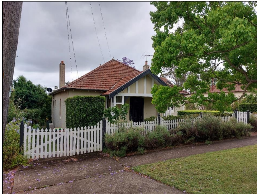
Figure 11 – Adjoining dwelling to the east at 29 Campbell Street
