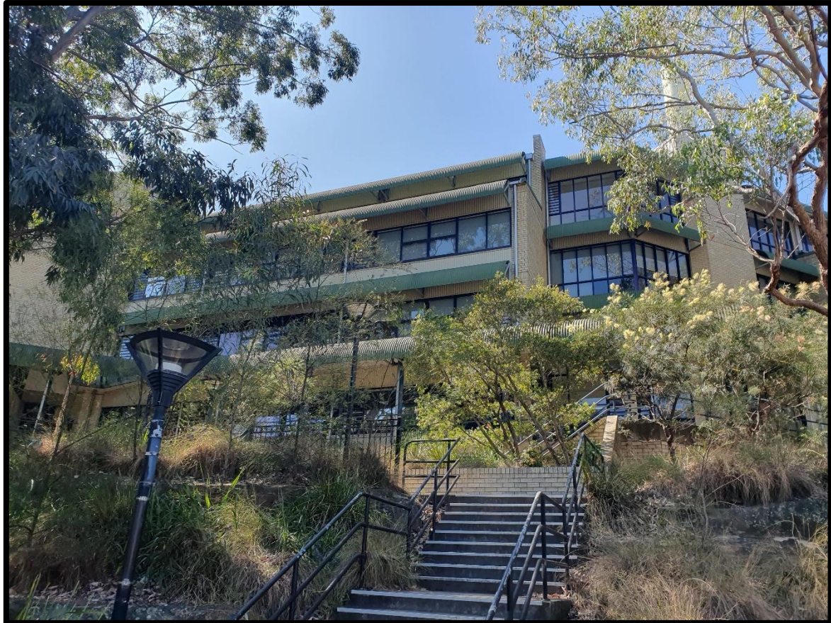
Figure 7- TAFE NSW Meadowbank campus to the north of the subject site as viewed from Constitution Road.
