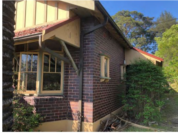
Figure 6 – View of the side elevation
