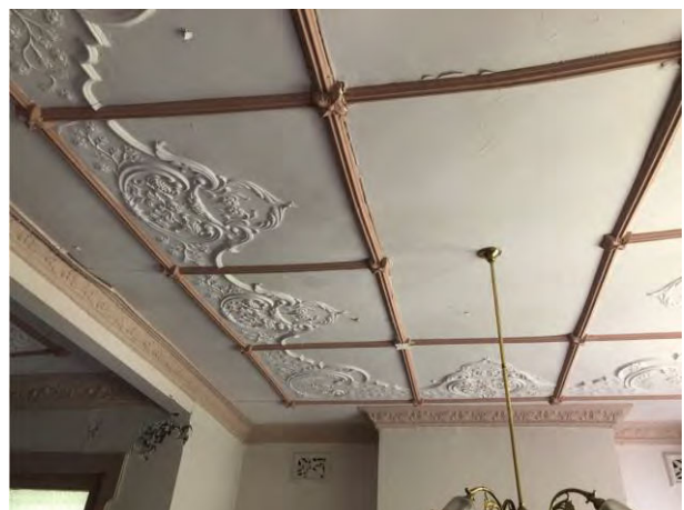
Figure 10 – View of the living room ceiling
