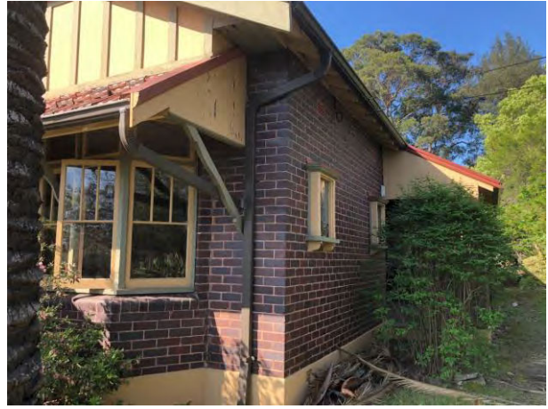
Figure 6 – View of the side elevation
