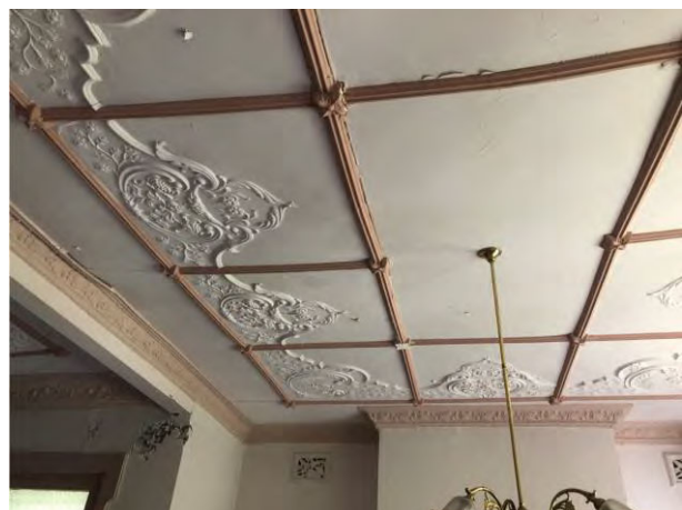
Figure 10 – View of the living room ceiling
