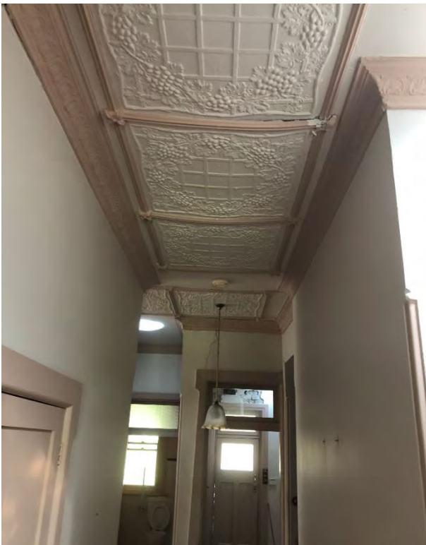
Figure 13 – View of hallway ceiling Source: Urbis
