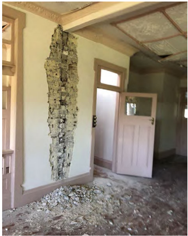
Figure 14 – View of wall in living room Source: Urbis
