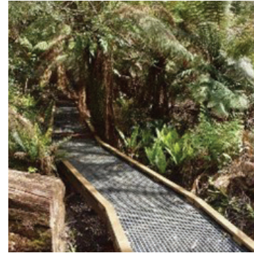
Accessible boardwalk and creek crossing with kick rails.
