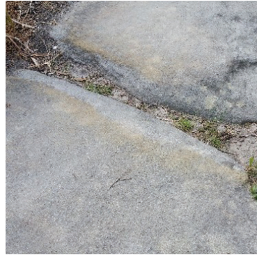
Track features - stormwater management using a drain cut into insitu rock.
