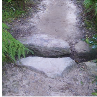
Track features - rock lined box drain / gutter.
