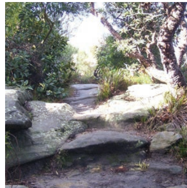
Track features - use natural rock platforms for stepping and infill with site stone to create a traffic-able track.
