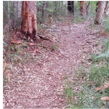
Track features - typical grade 3 track with compacted earth surface.
