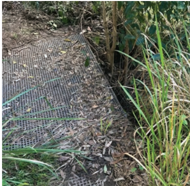
Track features - mesh deck panel across minor drainage line.
