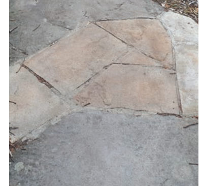
Track features - stone flagging where pavement hardening or infill is required.
