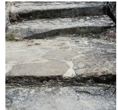
Track features - infill stone flagging and rock leveling to create a passable track over insitu rock outcrops.
